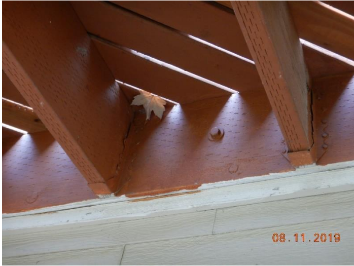
The deck is lag bolted to the home
