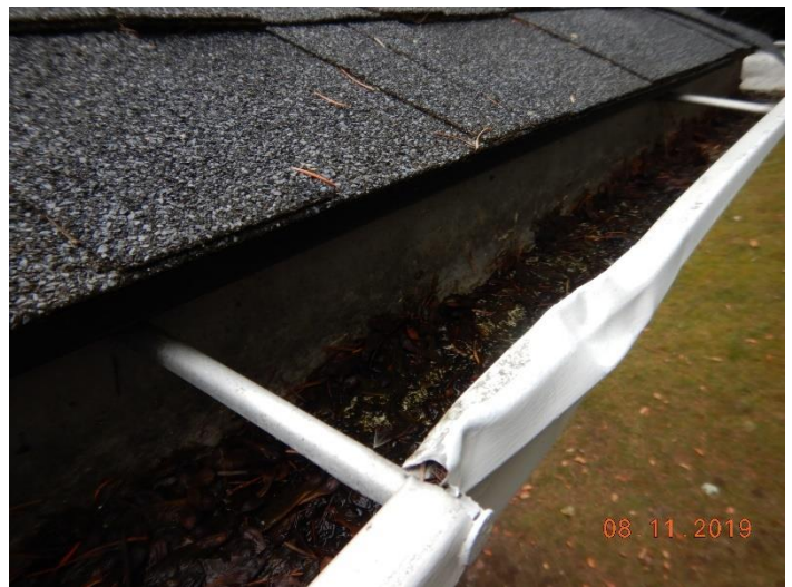
Dented gutter
